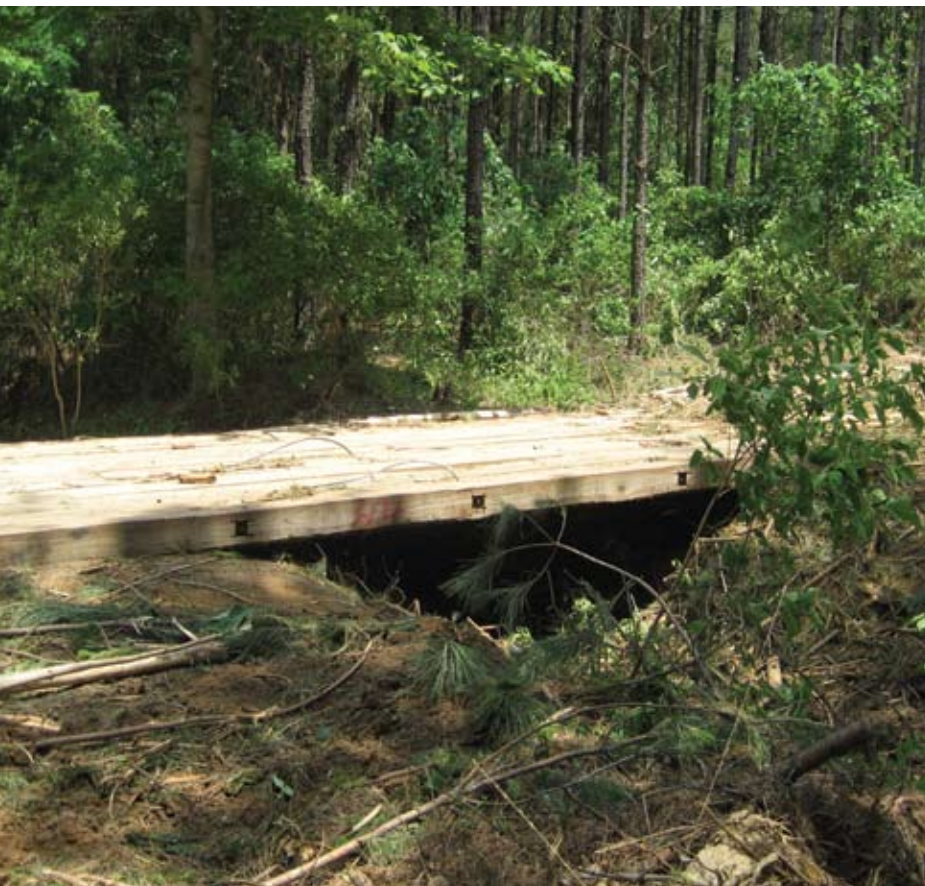
Here's an example of a bridge used to skid timber over a creek crossing. This particular bridge is 24-feet long and is made from hickory and red oak.
